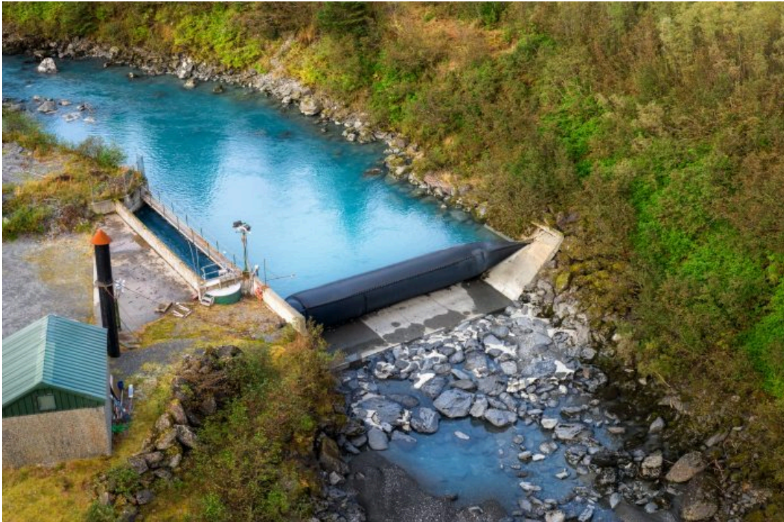
Power Creek hydroelectric plant, seven miles east of Cordova. Photo courtesy of Cordova Electric Cooperative
