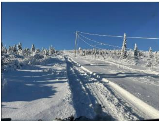
One of the projects includes relocating transmission-line poles that run through permafrost-ridden areas, to keep them poles from sinking.
